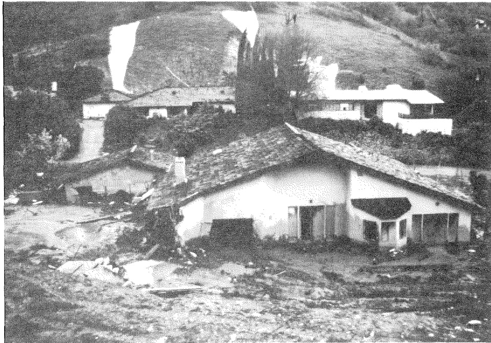
FIGURE A18 Rear yard and house of a pre-1963 subdivision inundated by mudflow off a natural slope during a 1980 storm in Tarzana, California. (Figure 4, James Slosson and James Krohn, Section 5.)
