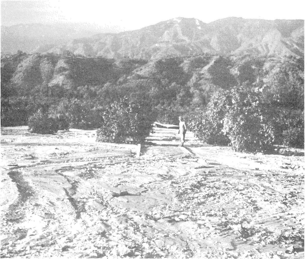
FIGURE 5 Concrete flood channel on an alluvial fan in Monrovia, completely filled with sediment in the 1938 flood (only a short length of the very tops of the channel walls is visible). Without an upstream debris basin a channel like this is useless in a flood.
