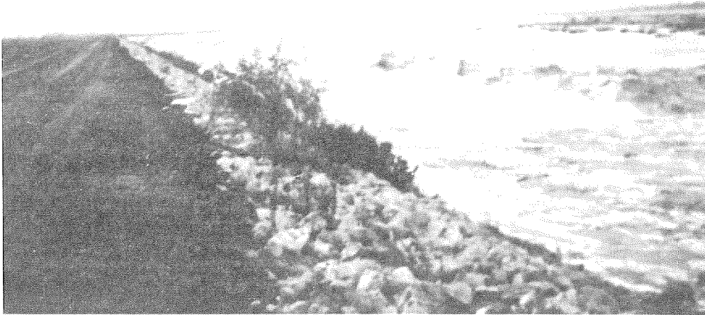
FIGURE A8 Impingement of flow on Santa Maria River levee. Damage or failure may start at points of attack like this. (Figure 5, James Stubchaer, Section 4.)
