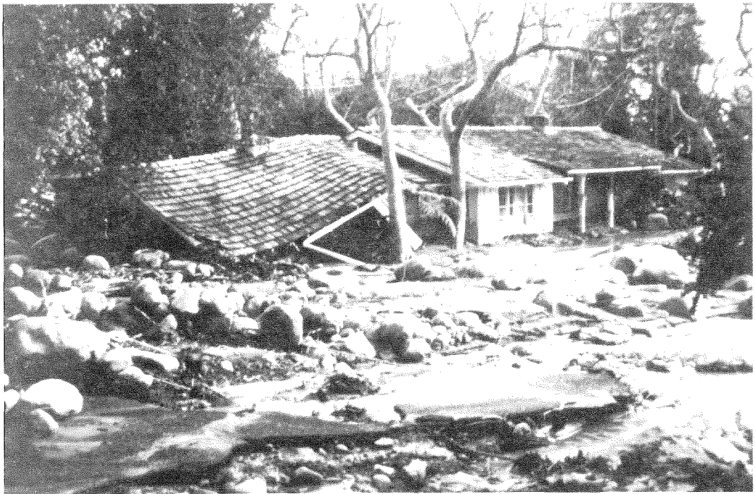
FIGURE A15 Damage from flood resulting from rain on a recently burned watershed. (Figure 10, James Stubchaer, Section 4.)
