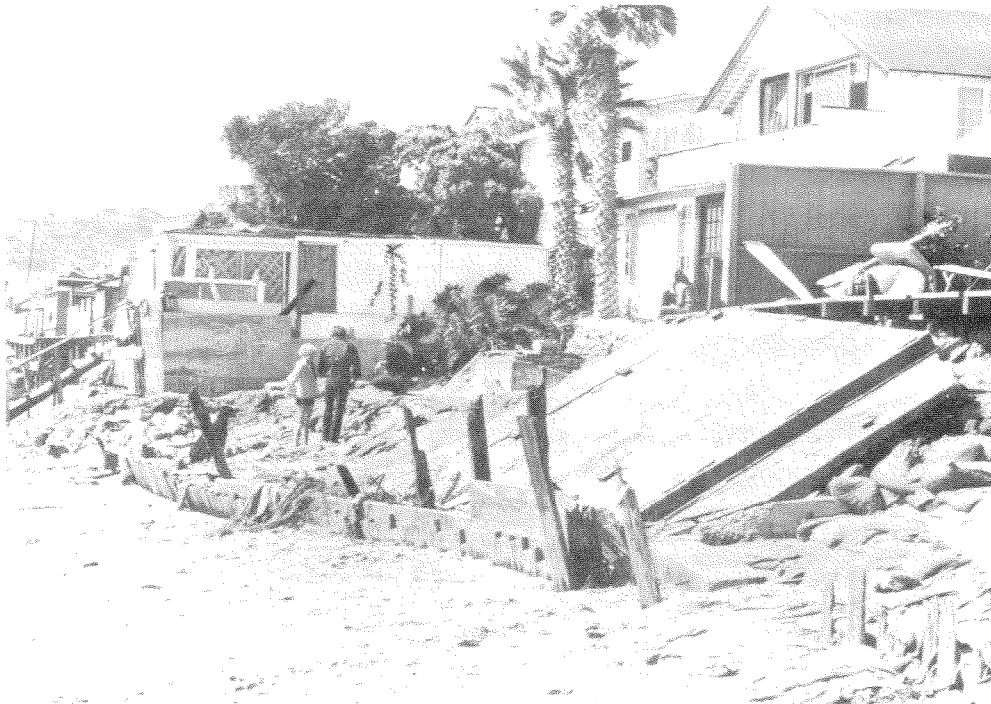
FIGURE A23 View up coast of damaged patio and destroyed bulkhead at lot 42 of Malibu Colony, March 7, 1978. (Figure 6, George Armstrong, Section 7.)
