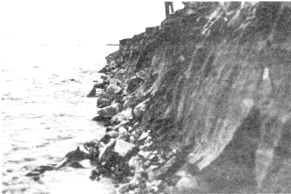
FIGURE A11 Eroded levee toe on the San Jacinto River (looking upstream). (Figure 6, Kenneth Edwards, Section 6.)
