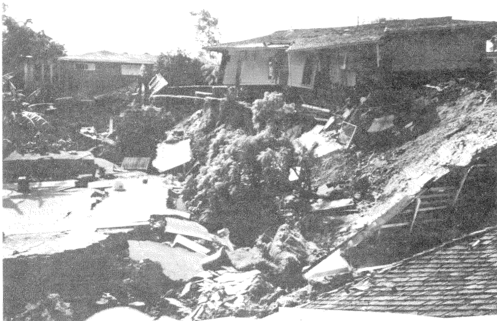
FIGURE A20 The Bluebird Canyon landslide (in October 1978) damaged or affected more than 50 homes in a hillside development in Laguna Beach. (Figure 1, James Slosson and James Krohn, Section 5.)
