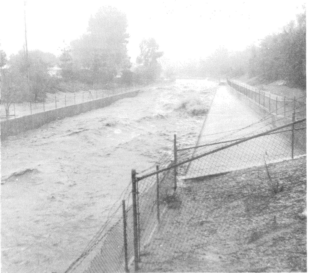
FIGURE A5 Some lined flood channels in the Los Angeles area flowed near their capacities, as shown in the view looking downstream on the Los Angeles River near Kester Avenue (approximately 1 mile downstream of Sepulveda Dam) on February 16, 1980. Note the standing wave resulting from side weir overflow. Photograph courtesy of Los Angeles County Flood Control District. (Figure 10, Joseph Evelyn, Section 3.)
